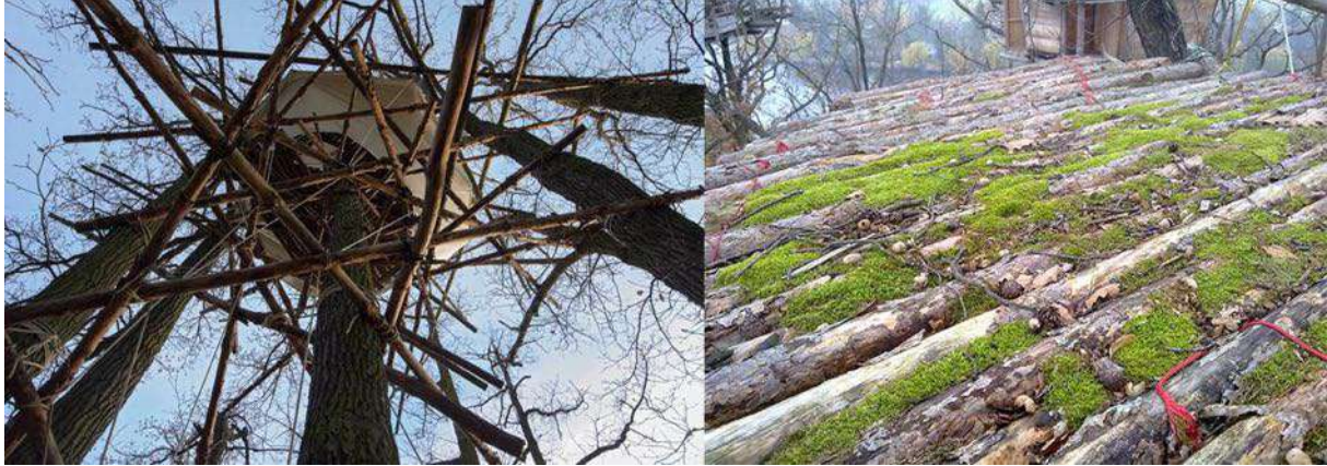
Figure 14: SpiralTreeHouse with self-standing flexible structure that is co-designed with wind and the tree to which it is attached. The platform on the right is being co-designed by the habitation of moss, providing comfortable flooring and mattress for humans and other species, thus extending present landscape. (photos: Zapletal 2014, Davidová 2012).
