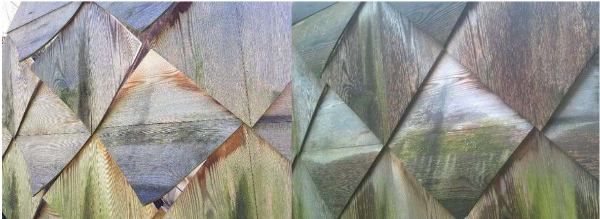
Figure 6: Ray 2*2013 Responsive Wood Envelope Prototype a) in semi-dry June 2018 weather when the screen is open for boundary exchange between exterior and semi-interior; b) after April light rain in 2017 when the system is closed, not allowing the humid and cold air to pass through the boundary; both after five and four years respectively of being exposed to weather and biotic conditions. The prototype got inhabited by Blue Stein Fungi, Algae and Lichen. These, namely the algae, are regulating the moisture content of wood, thus co-causing its warping. Notice also the organisation of algae habitation caused by the material's fibre direction and position within the design that is affected by material performance and form. Thus it is organised through its moisture and the organism's abundance and distribution interaction (Davidová, 2017a). (photos: Davidová 2017 - 2018)
