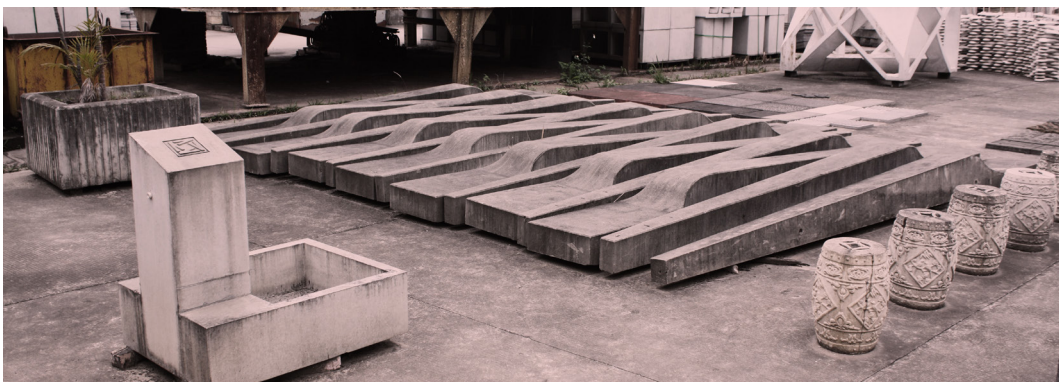
Figure 7.54: Pre-cast concrete landscape elements in Vanke's Housing Industrialization Research Center in Dongguan (source: picture by the author).
