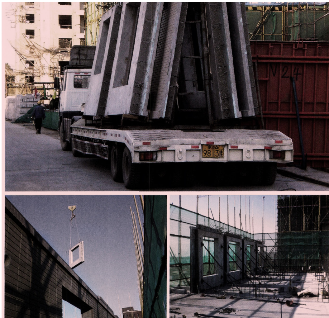
Figure 6.6.7: Pictures of prefabricated construction elements and construction site of Beijing Vanke COFCO Holiday Town (Source: Fan Zesen, Du Peiwei, & Du Jua, 2011).
