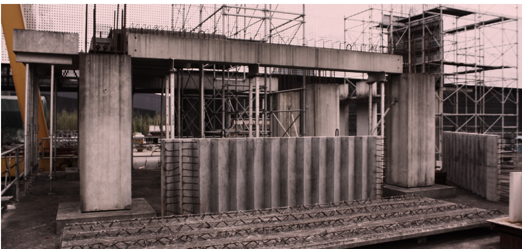
Figure 7.46: Prefabricated concrete elements in Vanke's Housing Industrialization Research Center in Dongguan (source: picture by the author).
