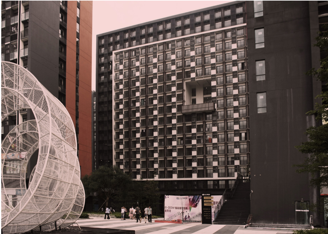
Figure 6.8.11: Central Plaza of Guangzhou Vanke Cloud City Phase 2 (Source: picture by the author).
