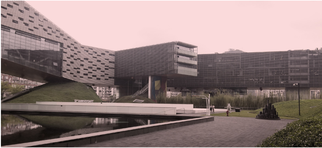
Figure 7.36: Vanke's headquarter in Dameisha, Yantian District, Shenzhen (source: picture by the author).
