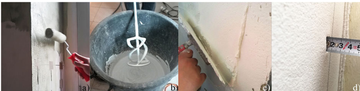
Fig. 5. a. Primer application. b. Mixing. c. Coating application. d. Final thickness.
