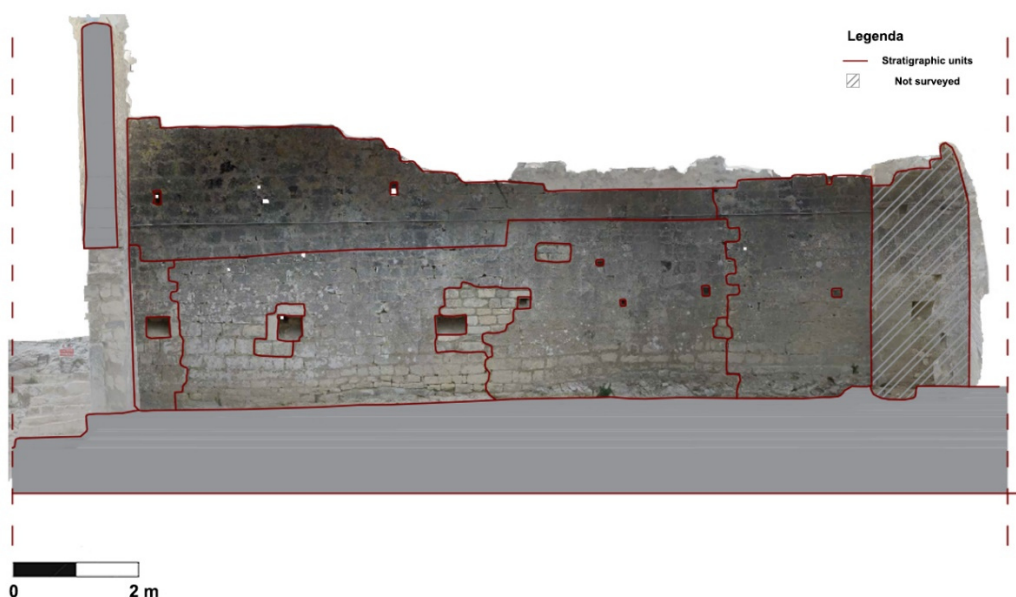
Figure 164 Rocca San Silvestro, dataset 1. Stratigraphic analyses of the west wall of the church (source: Arrighetti, 2017) reported on the orthophoto generated from the Freedom 360 system
