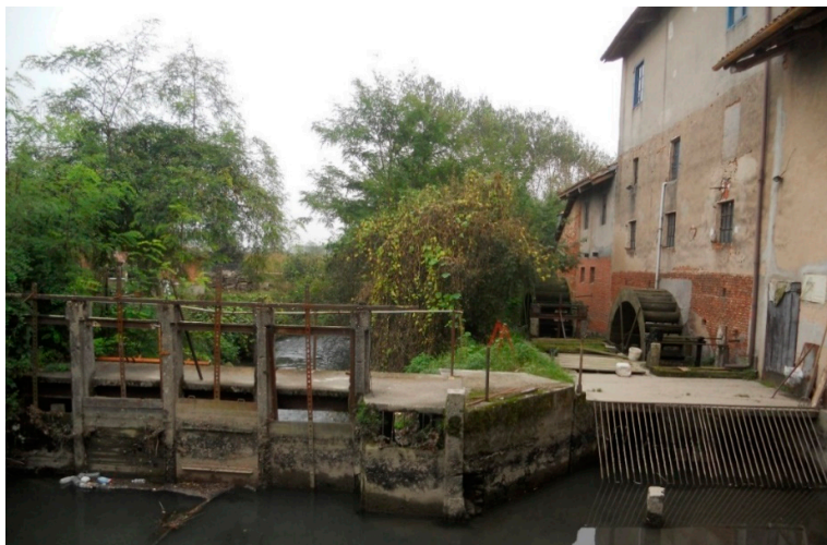
Figure 3. Forno mill: The water inlet and the two water wheels.
