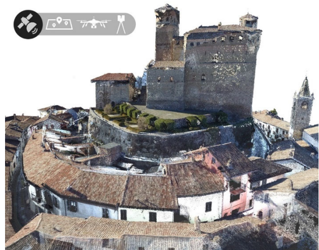
Figure 2. Point cloud obtained by geomatic survey
