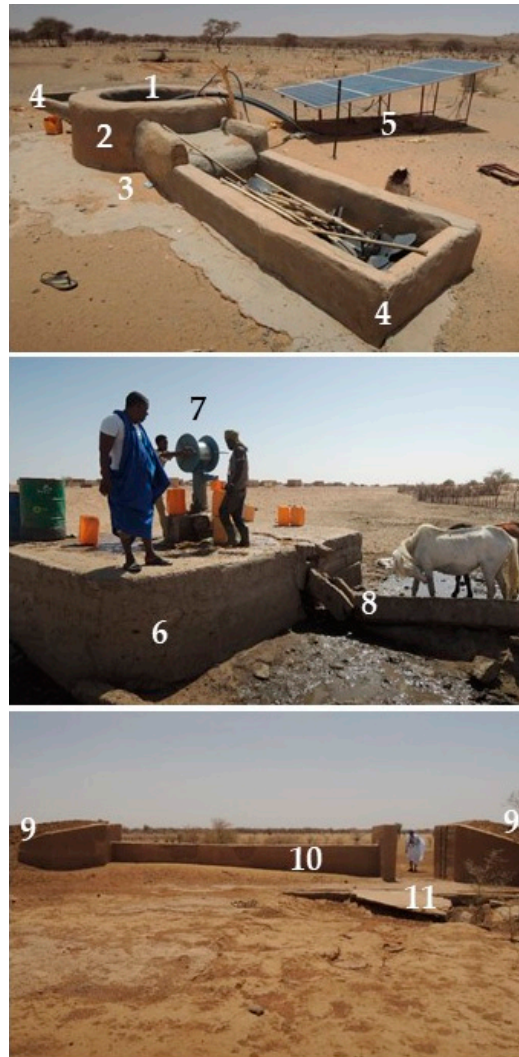
Figure 12. Open well (1) showing low apron (2) and basement (3), water trough for cattle watering (4), solar panels (5) in Boukhzama 1; a well provided with raised basement (6), a manual water pump (7), and a broken water trough (8); an earth embankment (9) provided with spillway (10) and lock (11) in Agoueinit.
