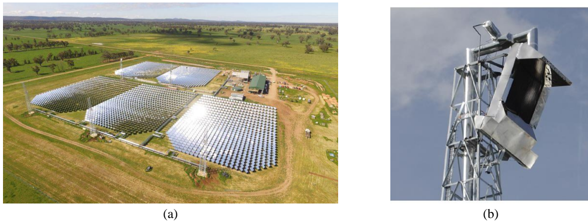
Figure 1 – Jemalong Solar Thermal Station, (a) aerial view of the whole plant and (b) solar receiver
