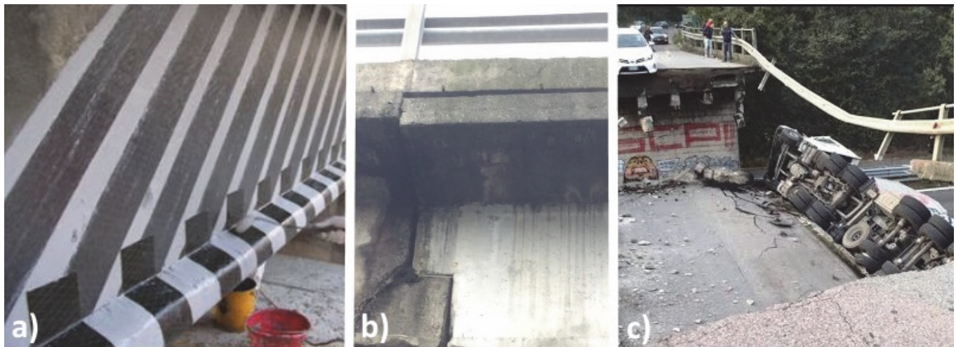
Figure 5: Dapped end corbel conditions before the collapse (a); humidity presence and water stagnation (b); failure loading configuration (c) [1].
