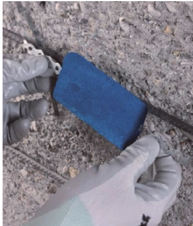
Figure 16: galvanic protection: sacrificial anode [Copyright: Mapei].
