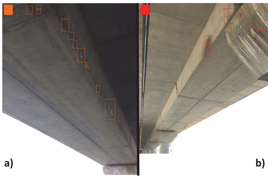
Figure 24: Detection of a Lv.3 damage (a); detection of a Lv.4 damage (b).
