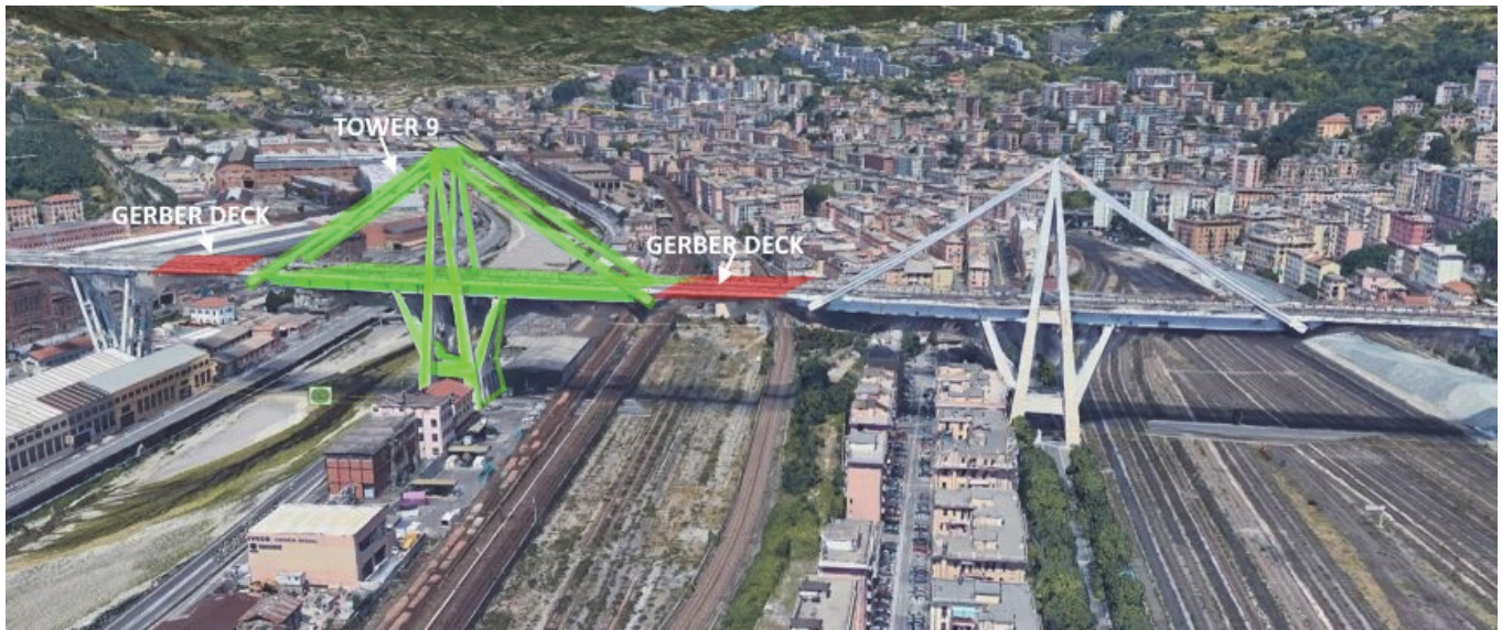
Figure 17: Involved structure in the collapse: tower and Gerber decks.
