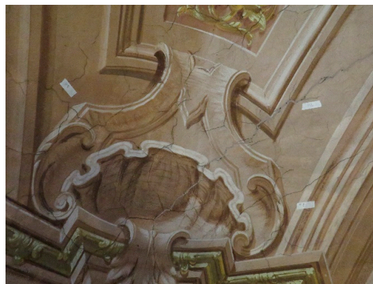
Figure 7. Survey area on the Pelagi room vault.
