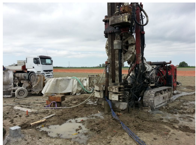
Figure 6. Installation of the instrumented micropile.
