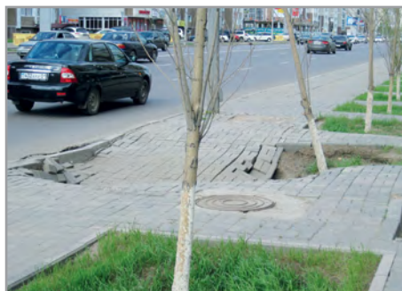
Subsidence in urban area induced by water network leakage. Credits: meadowsaffron on flickr
