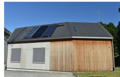
► Fig. 1: Exterior view of the ZEB Test Cells Laboratory, with the two cells on the left-hand side of the building.
