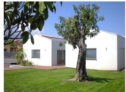
► Fig. 1: External view of the house
