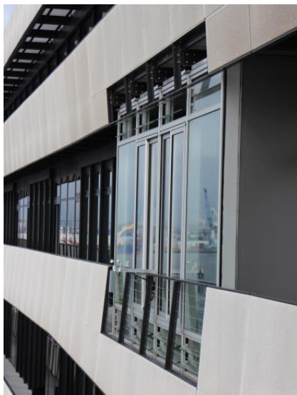
► Fig. 1: HCU Hamburg, South façade
