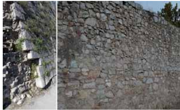
Fig. 13- Building the inner part towards the terreplein (right) and the internal part and scarpa (left) of the Contarini bastion (author)
