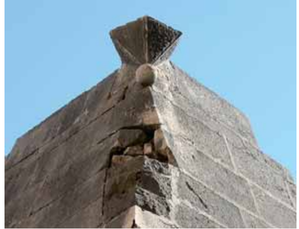
Fig. 9- Bottom part of a turret, bastion Priuli (author)
