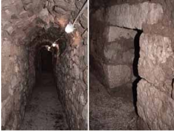
Fig. 7- Contramine gallery (on the left) and the entrance to the small room (right), eastern demibastion (author)
