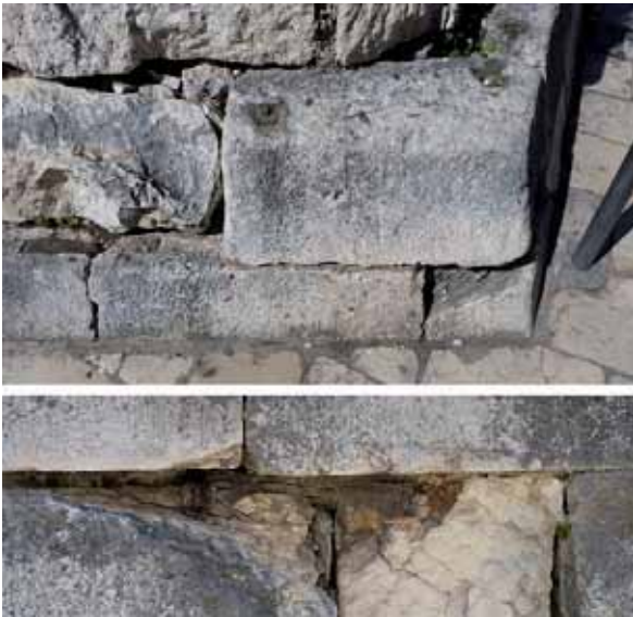
Fig. 11- Regular-shaped blocks (up) at the corners of the bastion, and the remains of cramps and lead (down), bastion Priuli (author)
