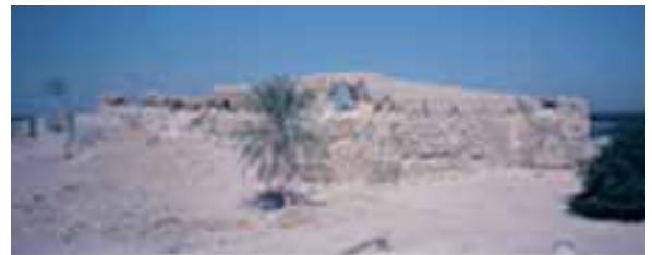
Fig. 3-4 (Campos, 2002) – Above, the land front with 2 bulwarks and the long curtain with the round bastion (1540) rehabilitated by Inofre de Carvalho (1558) and later replied at Bahrain. A ditch was here, from sea to sea. Bellow, the bulwark of the main gate, seen from the beach side, with posterior adding at the top
