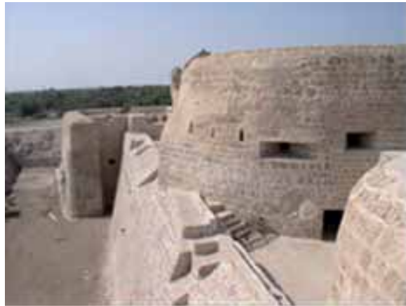
Fig. 10- The round bastion of the great South curtain and an orillion casemated bulwark at the corner of the ditch (Campos, 2005)
