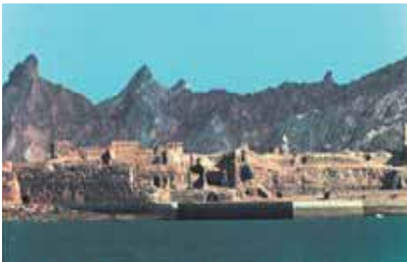
Fig. 1-2- Approaching the island by South with the ruins of the fortress (Campos, 2004). Bellow, model of the architectural survey of present condition (Campos, 2004)
