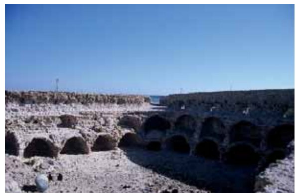
Fig. 6-7- (Campos, 2004) - Larak Fort, view from outside and inside, with posterior addition of constructive elements over the vaulted platform of terreplein of the fortification
