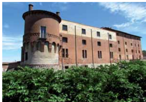
Fig. 1- Saluzzo Castle, view overlooking the hillside
