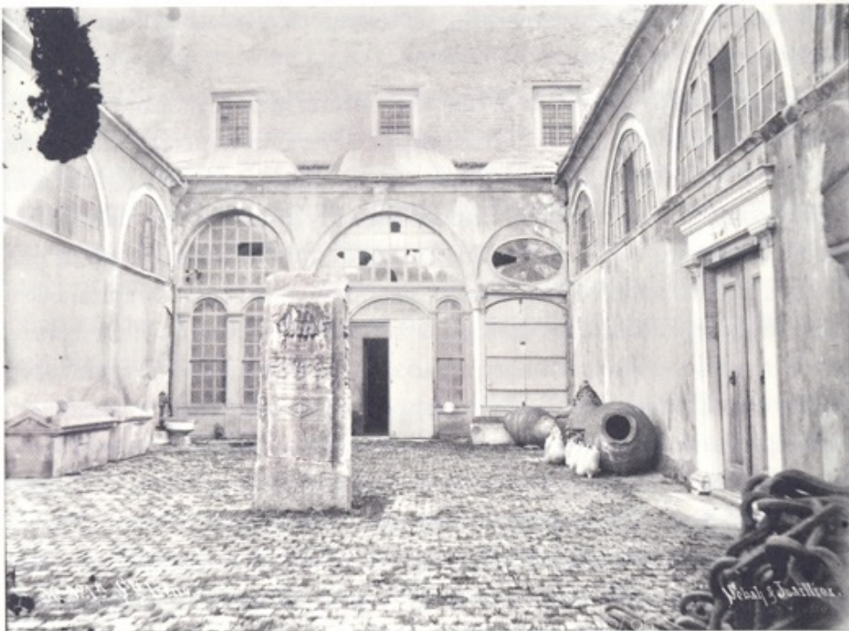
Figure 7: The courtyard of San Irene Church in the late nineteenth century. In Wendy M. K. Shaw, "From Mausoleum to Museum", p.428.
