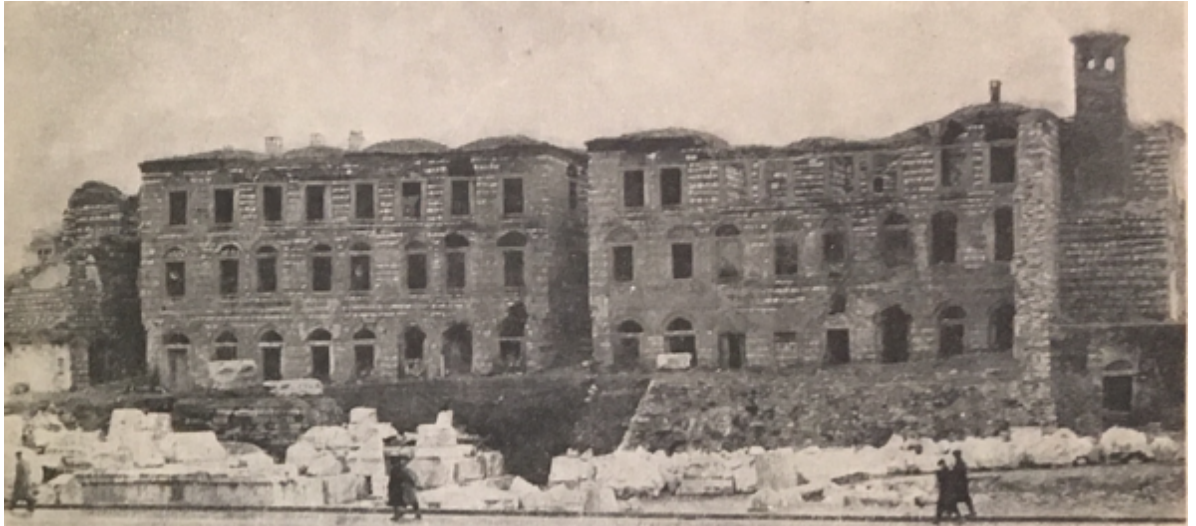
Figure 65: the Simkeşhane after deconstruction. The findings in the courtyard remained on the sidewalk after the buiding was half-demolished. In -, Rölöve . 551
