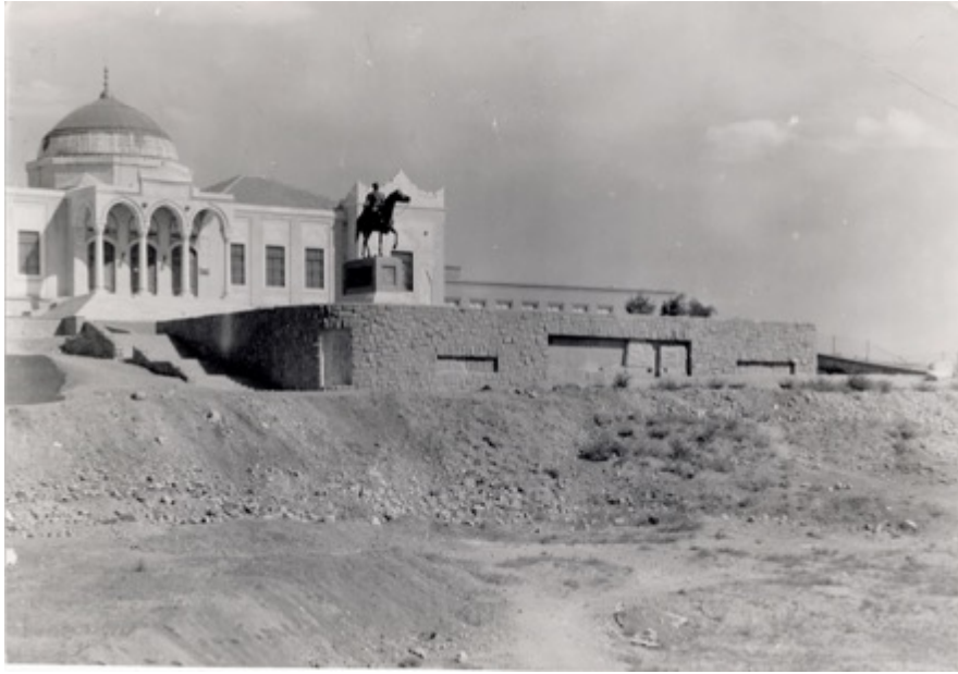
Figure 42: Ethnography Museum during construction. SALT Online Archive, TASUH6814 .
