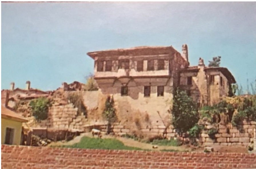
Figure 71: Arslanlu House in Milas before registration. In Azra Erhat, “Anıtlar”.
