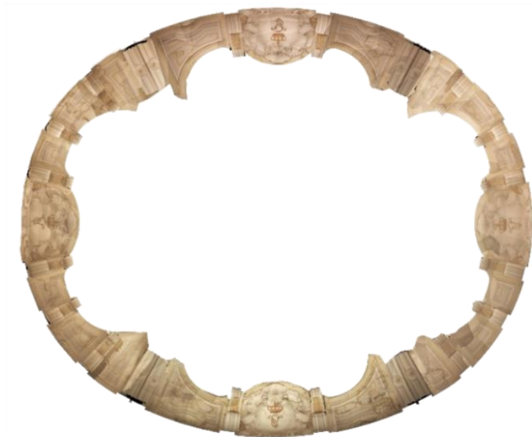
Figure 17. Orthophoto of the intrados of the balcony of the Stupinigi royal residence hall of honour, generated by SfM methods.
