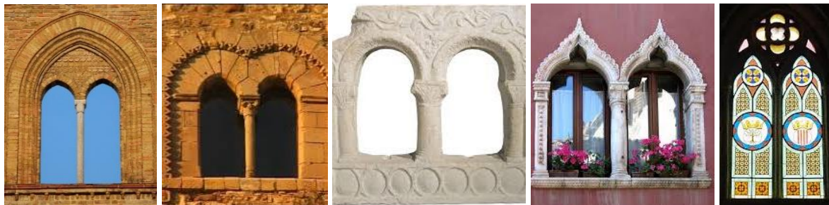
Figure 11. Schema of a gemel window and a series of images of windows which respect that schema.
