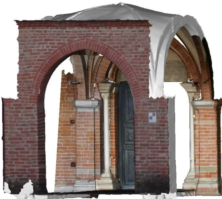
Figure 116. The bay further segmented in its parts (LOS 3)
