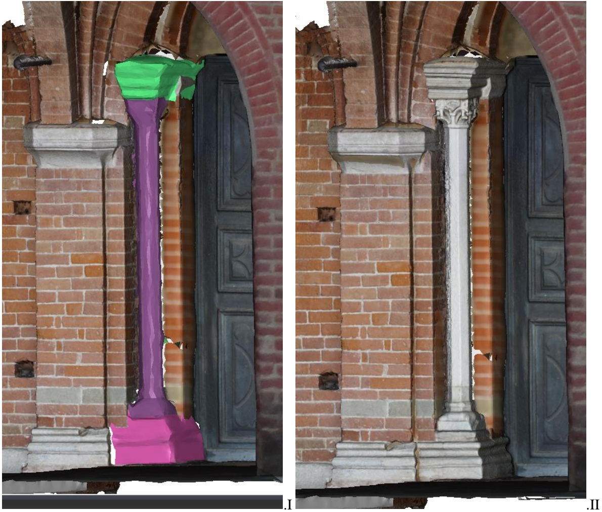
Figure 117. (I) The column is highlighted as it is segmented and represented in LOS 4; (II) The representation deriving from a further survey (realized with digital images processed in a structure-from-motion software) is integrated in the 3D model of the bay. It is realized for being segmented for LOS 5 - 6.
