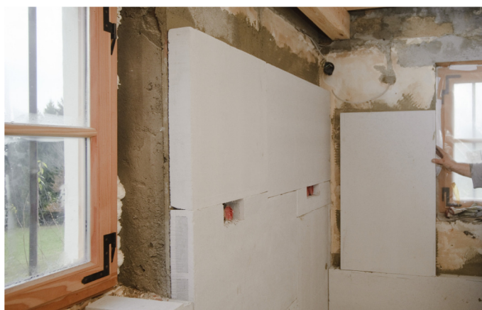
Figure 7: Fumed silica, coupled with calcium silicate panels [31]
