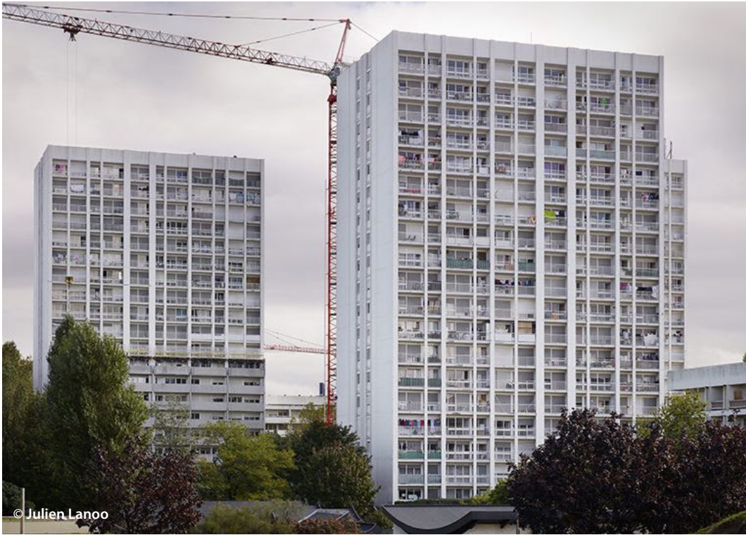
Buildings before retrofit
