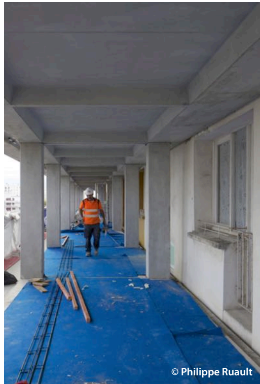
Top: Buildings before retrofit Bottom: Loggias under construction
