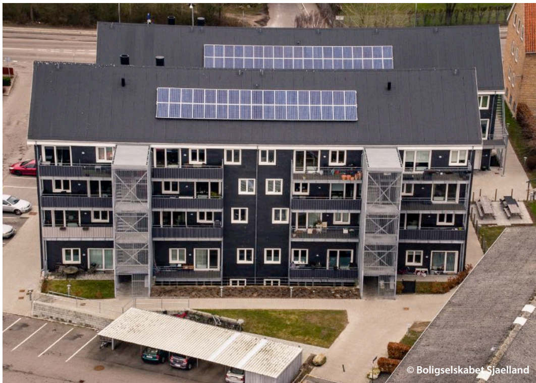
Top: Aerial view of Block A and Block B after retrofit Bottom: Block A rear elevation with added external stairs and balconies
