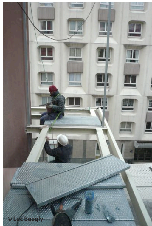
Top: Building before retrofit Bottom: Building during retrofit (balcony flooring structure)
