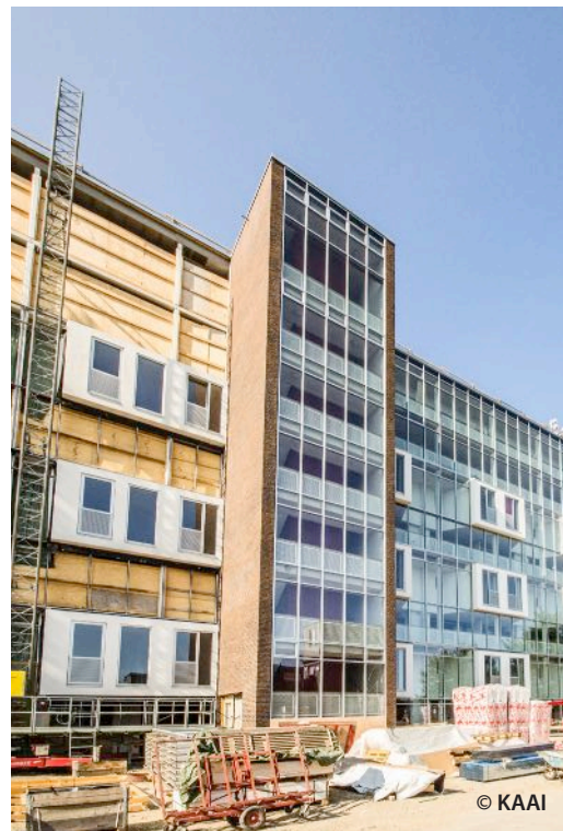
Top and bottom right: Building during retrofit Bottom left: Project sketch
