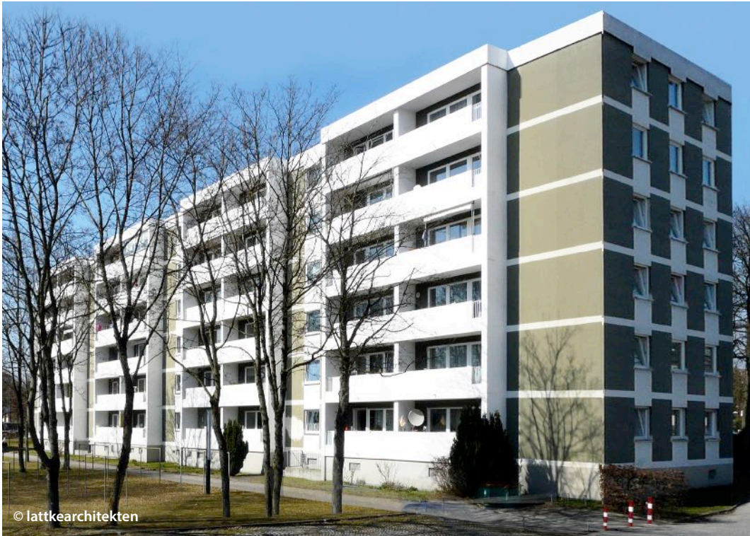
Grüntensstraße 34-36, building before retrofit
