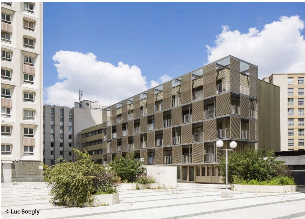
Building after retrofit Different treatment of the façades
