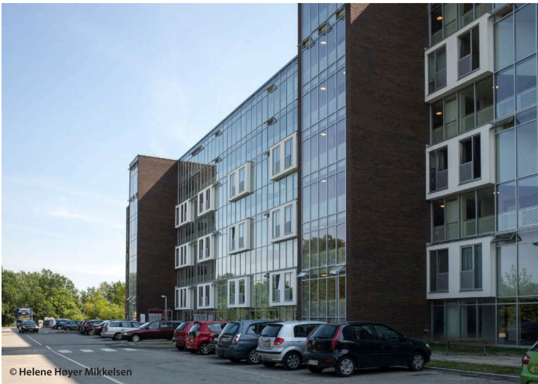
Building after retrofit Exterior of the north façade with added stair and elevator towers
