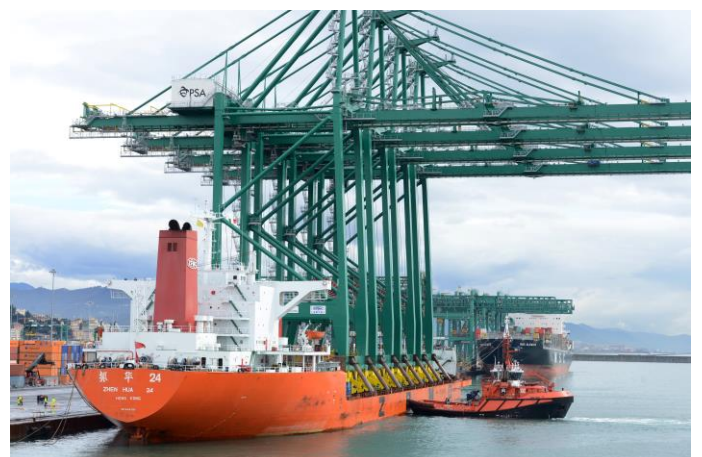
Figure 3. VTE’s quay gantry cranes - gooseneck type
