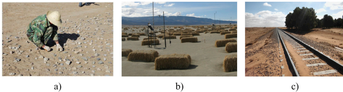
Fig. 16. Unstructured Hedge system: a) gravel surface (reprinted from: Liu et al., 2011, with the permission from Elsevier), b) large roughness elements (reprinted from: Gillies et al., 2015, with the permission from Elsevier), c) trees planted over dunes near a railway.
