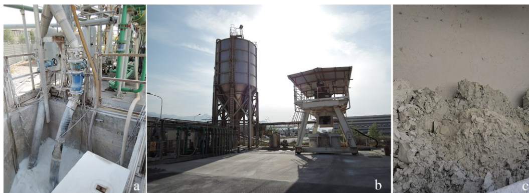
Figure 31: a) pumps sending waste water of stone cutting/finishing processes to the filter-press plant; b) filter-press plant; c) slurried extractive waste after the treatment.
