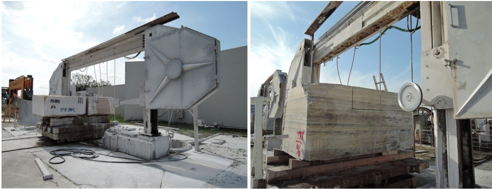
Figure 20: squaring/cutting of stone blocks with mono diamond wire technology
