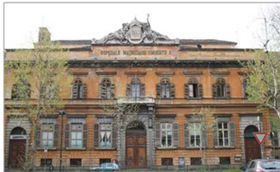
Figure 7.1 Umberto I, Mauriziano hospital in Turin.
