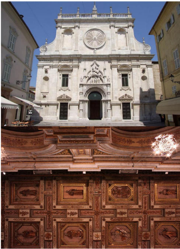
Fig. 4 The case study B: the Basilica of San Nicola, main façade (top) and the coffered wooden ceiling (down). Source: http://www.iluoghidelsilenzio.it/ and authors
