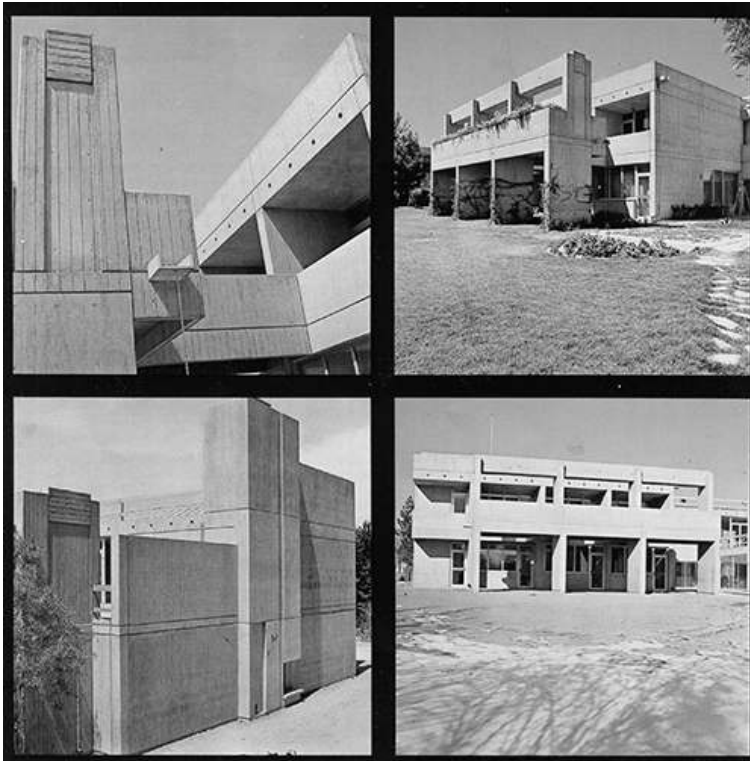
Figure 6: Views of the ambassador's residence.
