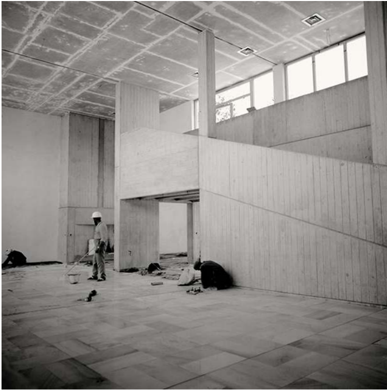
Figure 10b: The residence's interior: view of the stairs leading to the ambassador's office.
