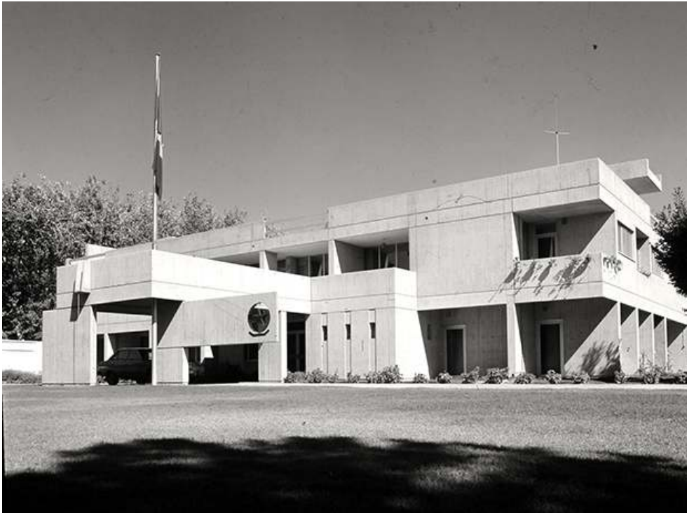
Figure 4: Overall view of the ambassador's residence.
