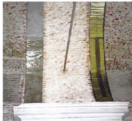
Figure 34: Complesso di Venaria Reale (TO) – Strengthening intervention with strips placed to the intradox and extrados of the vaults. Source (Credali, 2002).
