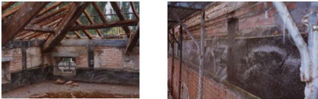
Figure 29: horizontal and vertical CFRP kerbs on internal and external walls. Source (Credali, 2009).
