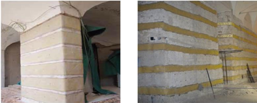
Figure 35: strengthening intervention with FRP in Villa Reale in Monza (sx), and Real Albergo dei Poveri a Napoli (dx). Source (Olympus, 2016) and (ResinProget, 2012).
