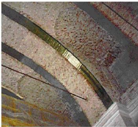
Figure 34: Complesso di Venaria Reale (TO) – Strengthening intervention with strips placed to the intradox and extrados of the vaults. Source (Credali, 2002).
