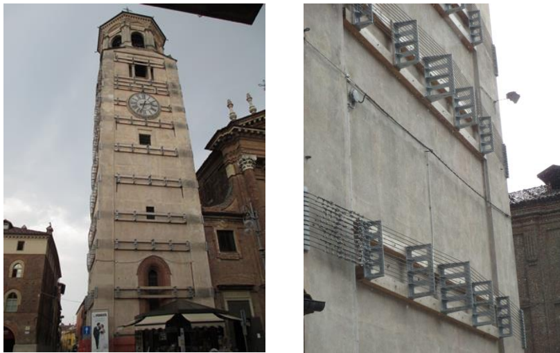
Figure 88: the belfry of the Fossano Cathedral with the strengthening intervention.
