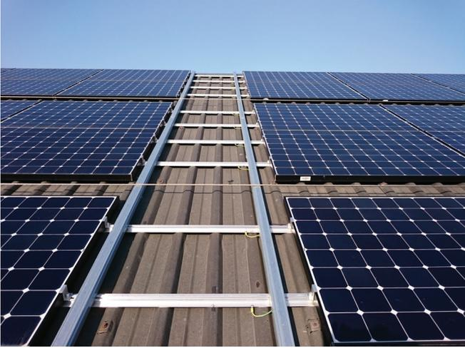
Fig. 3. PV modules, aluminum frameworks and bonding conductors.
