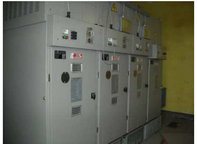
Fig. 5. MV switchgear in the faulted substation.
