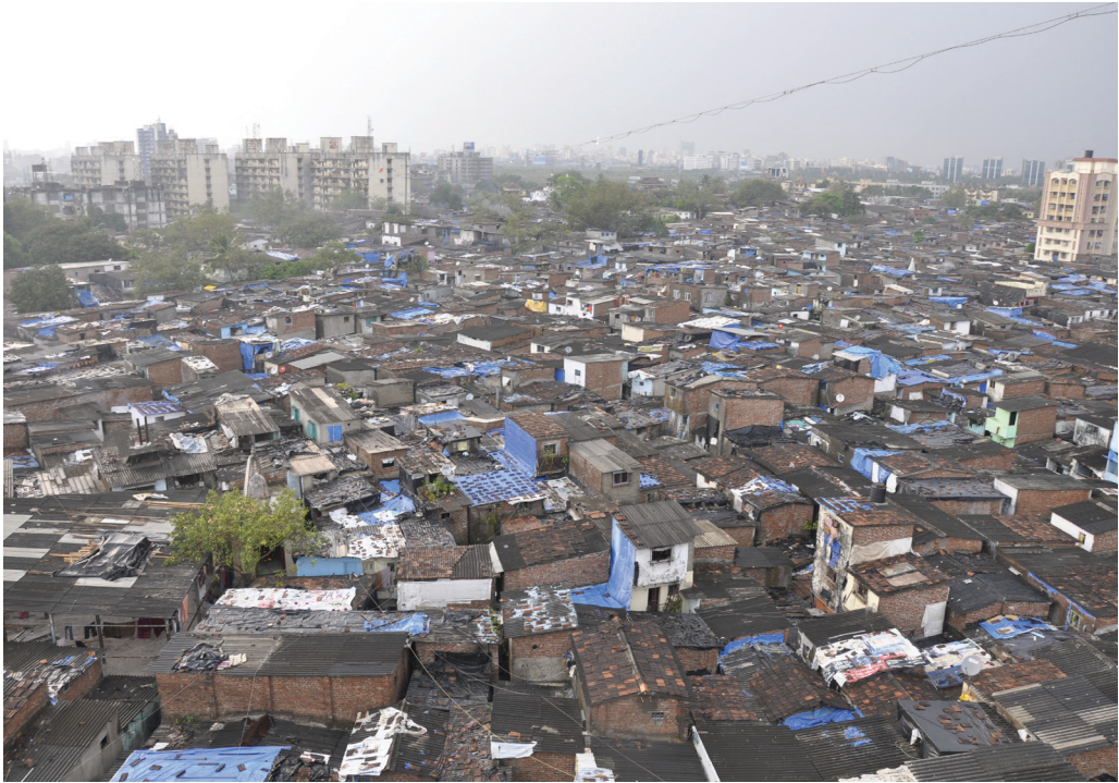
FIGURE 1: View of Dharavi.
