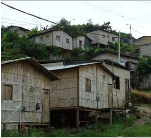
1 The poorest part of the informal 'El Fortin' neighborhood, 'La Cordillera del Condor' The image shows a "tricycle", one of the most popular vehicles used in informal settlements. The poorest houses are made of bamboo panels and clay bricks
