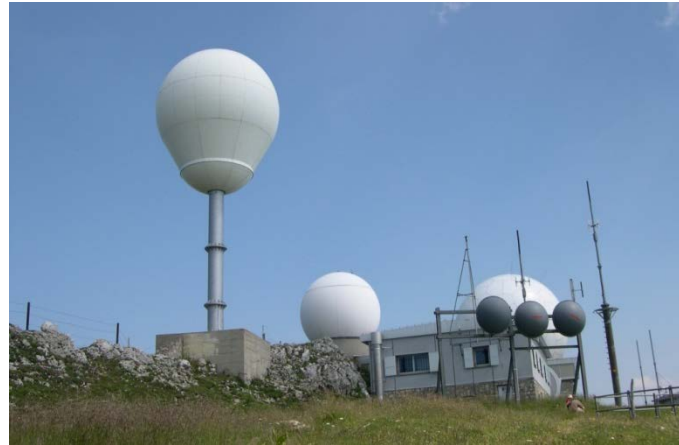
Figure 2.9 - Typical radar station for meteorological and civil purpose
