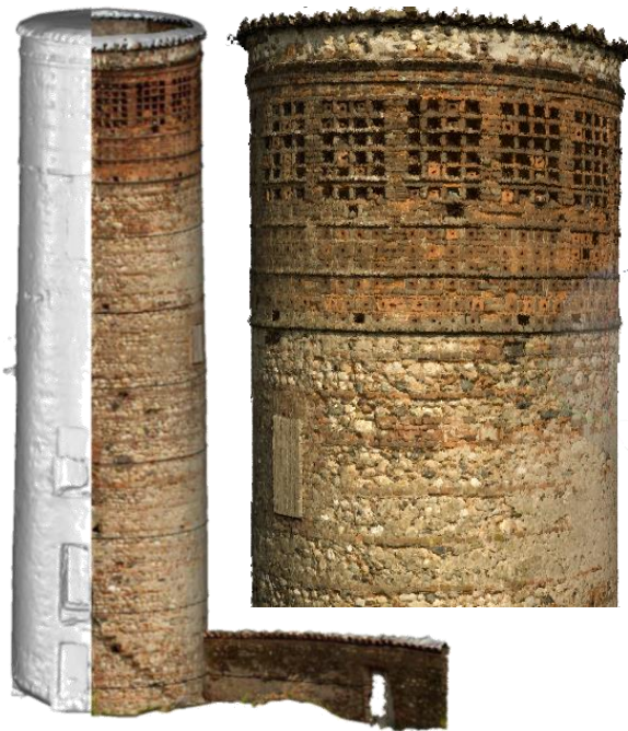
Figure 5. The 3D photogrammetric model and a zoomed image on the dense point cloud on the dovecot
