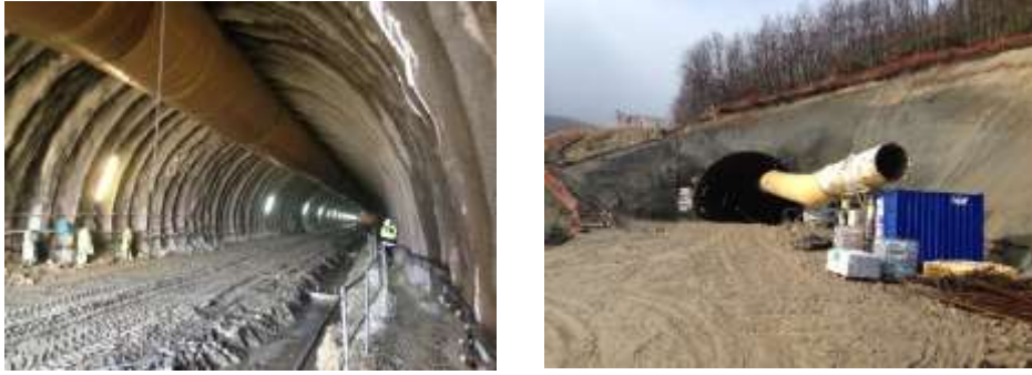
Figure 3.3: Excavation phase of the Padornelo Tunnel.
