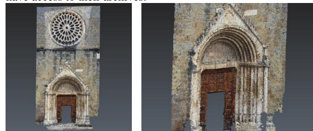
Figure 17. First test of point cloud generation of the portal before the earthquakes
