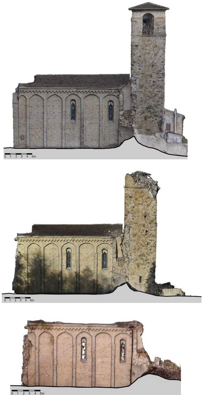
Figure 7. Orthophoto of East wall. Top: September (t1); centre: December (t2); down: January (t3)
