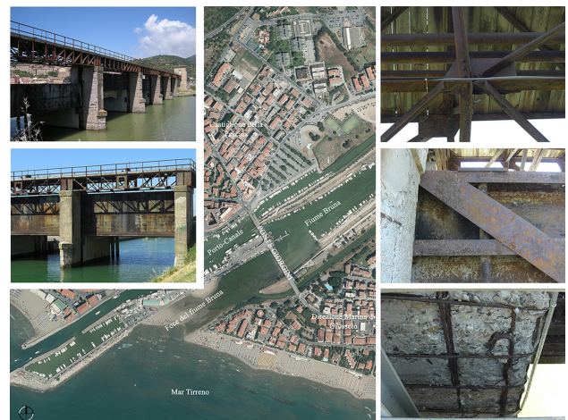
Figure 1. The Giorgini Bridge
