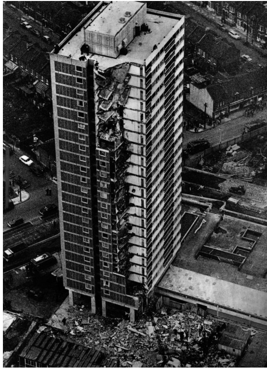
Fig. 2.2 Ronan Point progressive collapse, London (1968).
