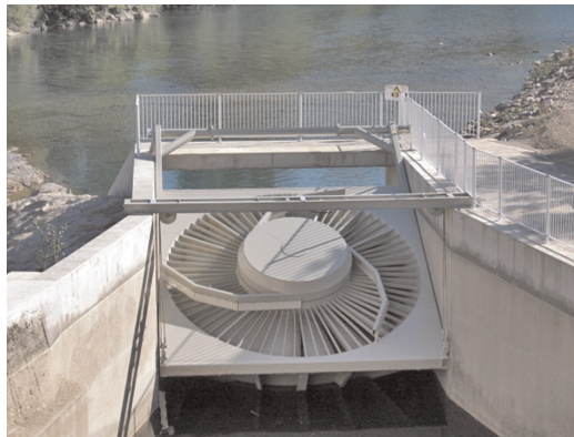
Fig. 1.5. The very low head turbine (Bozhinova et al., 2013).
