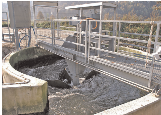
Fig. 1.7. The gravitational vortex converter (Bozhinova et al., 2013).
