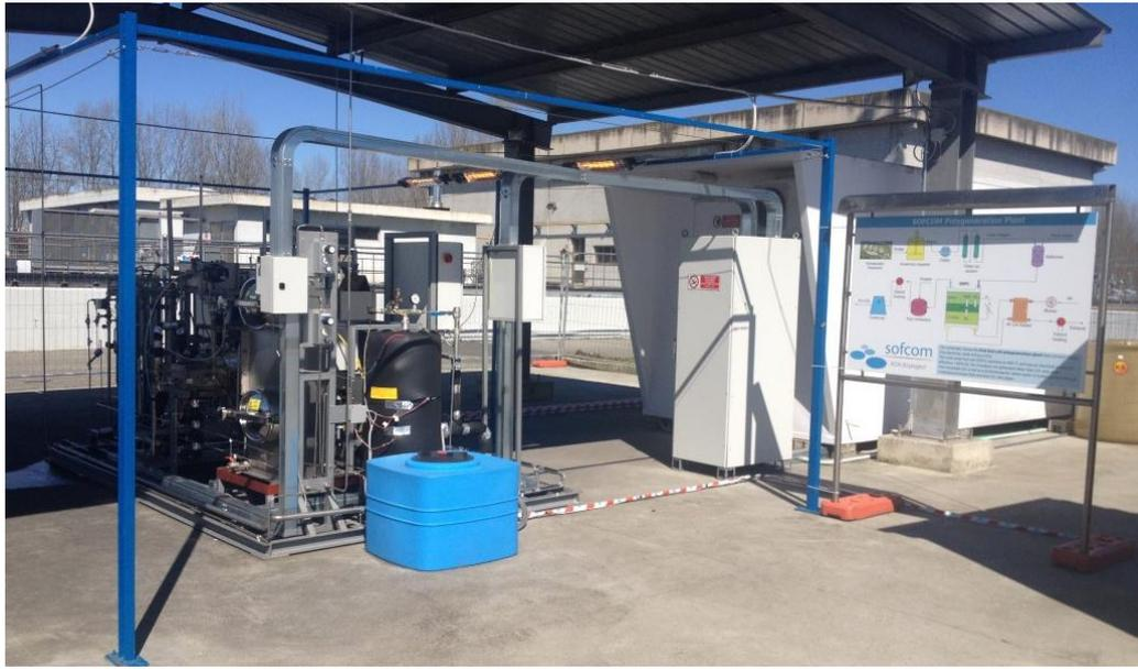
Figure 39. SOFCOM proof-of-concept at the SMAT Castiglione WWTP – from biogas to CO<sub>2</sub>.
