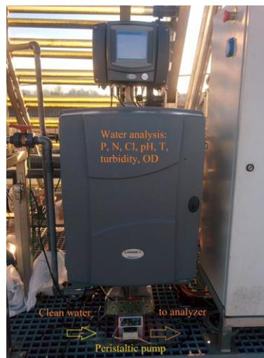
Figure 71. Wastewater analyzers.
