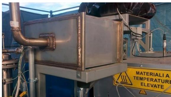
Figure 56. CHP water heat exchanger.
