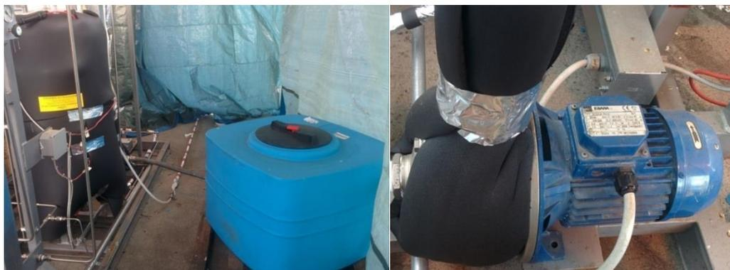
Figure 47. Atmospheric and Pressurized demi water tanks. Demi water pump to feed pressurized tank.
