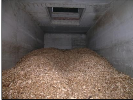
Figure 4.9 – Chips storage tank
