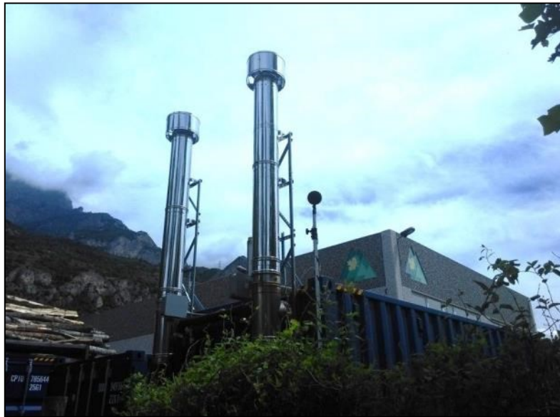
Figure 7.8 – Positioning of the measuring point relatively to the emission source
