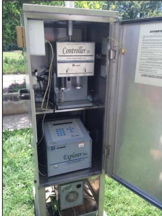
Figure 7.6 – Strumentation for the sampling of PM 10 concentration
