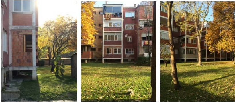
Figure 15: Enlargements of the buildings in the “Prolet” settlement, Skopje, 2015.
