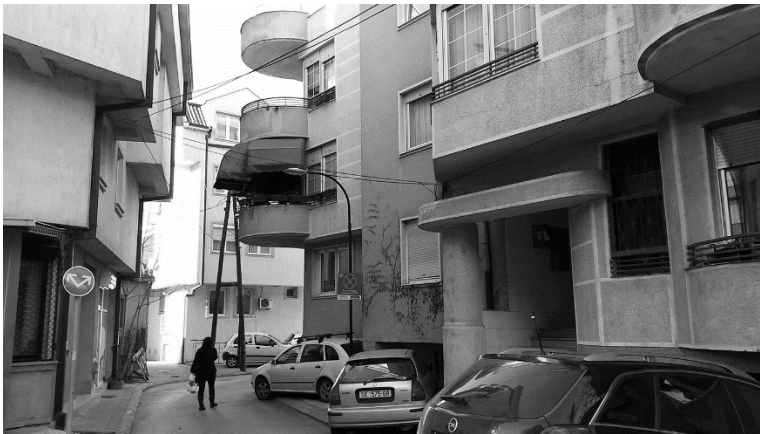
Figure 3: a typical street view in Debar Maalo depicting the consequences of uncontrolled densification
