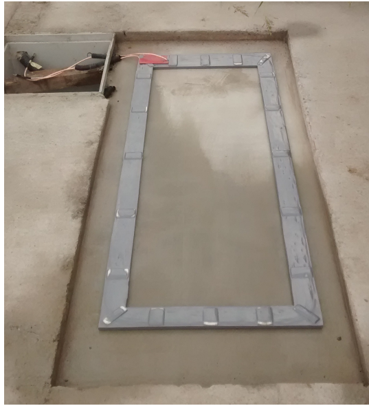
Figure 7.18: Coil L_2 inserted in the epoxy resin block placed on the concrete housing.
