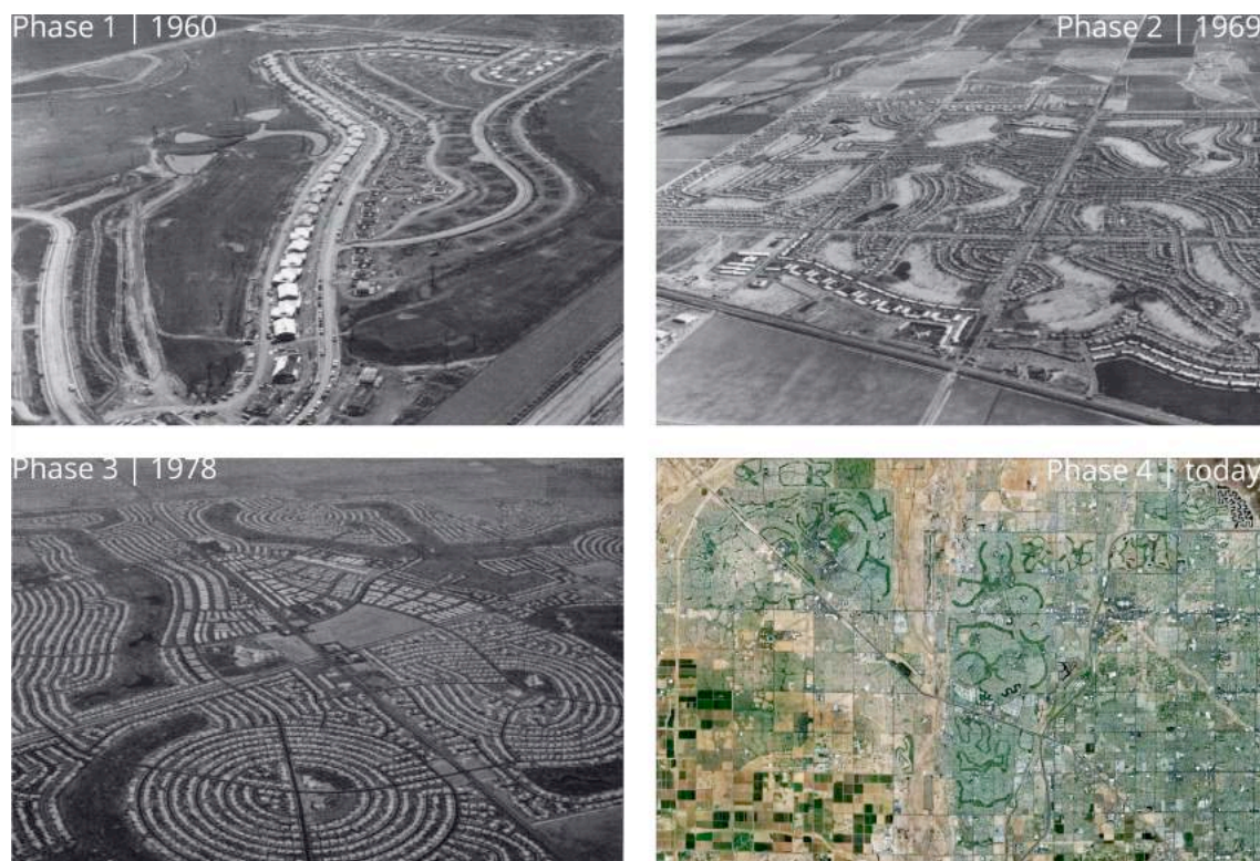
Figure 2. Sun City's the different phases of construction.
