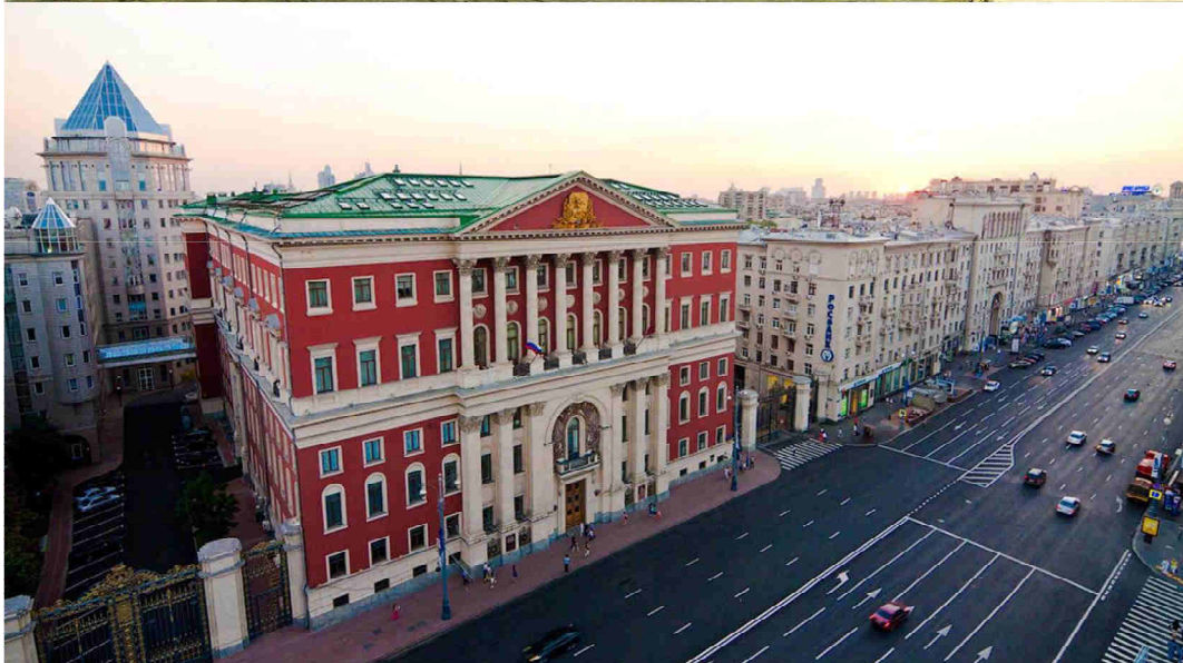
Fig. 4 - Chernyshev House, project by M.Kazakov. Now it is the building of the Moscow mayor's office.
