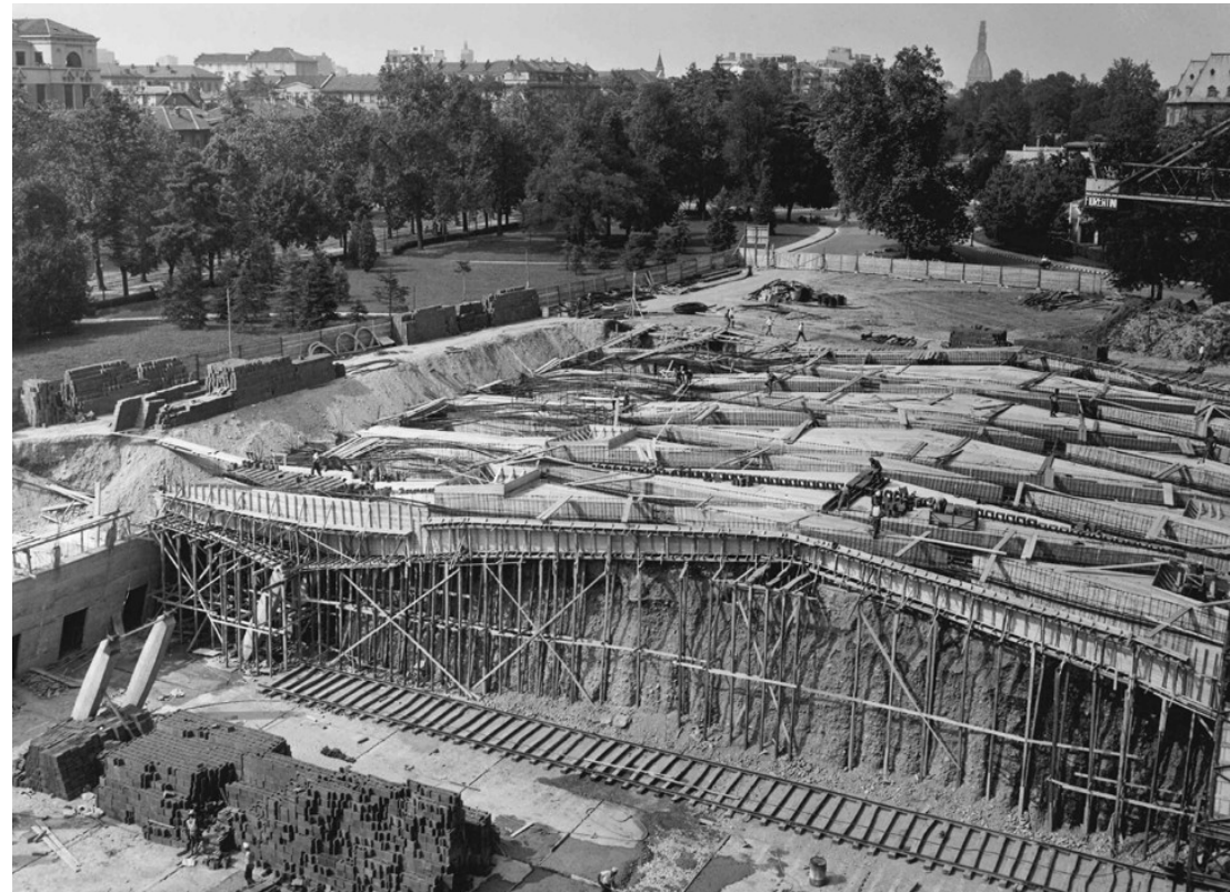
Figure 3 Building site image. Source: Luigi Ravelli's Private Fund. He was the planning supervisor at Servizio Costruzioni Fiat - at the time of construction of the pavilion [Bruno, 2013].
