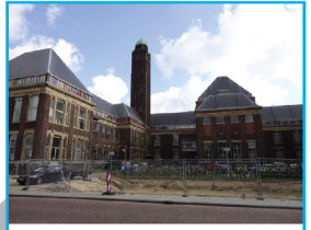
Faculty of Architecture Building 8
