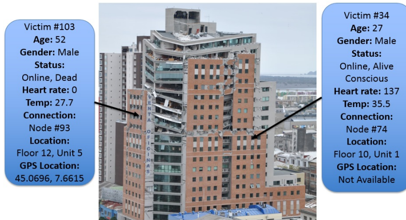
Figure 8: An example of the system application after earthquake.
