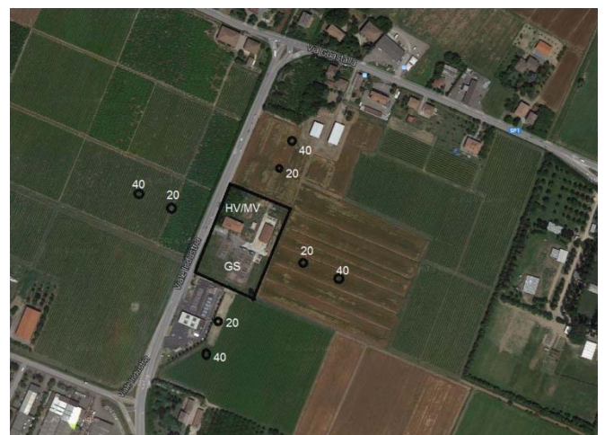
Figure 9. HV/MV substation situated in Carpi (Italy)
