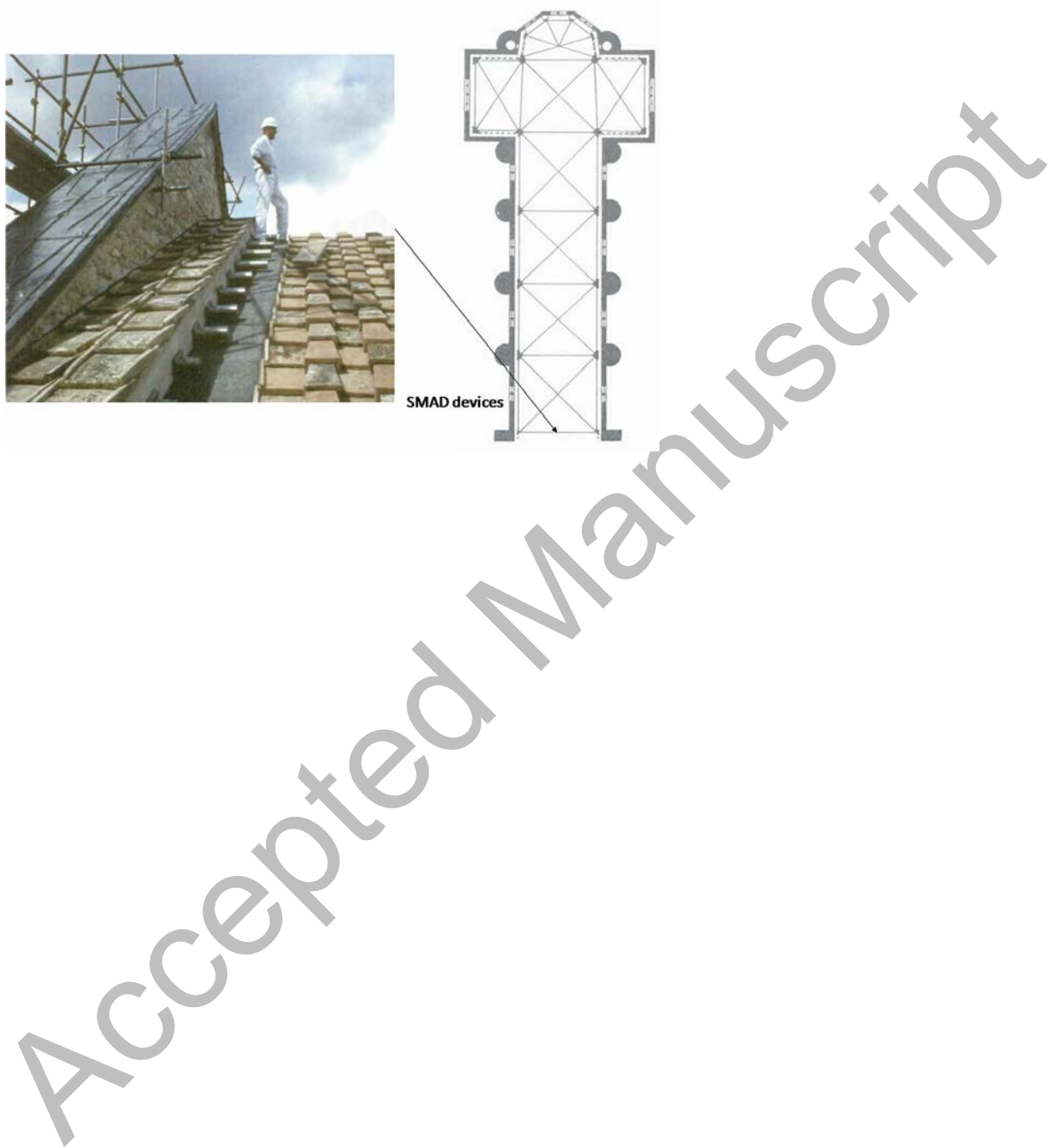
Figure 9- Installation of SMADs at the Tympanum-roof interface (Croci et al., 2007).
