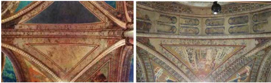
Figure 5- Restored Frescoes after 1997 Earthquake. a) Cimabue; b) Giotto vaults.
