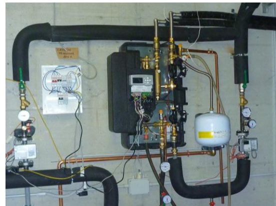
Figure 5 –FPC Pumping and heat transfer station
