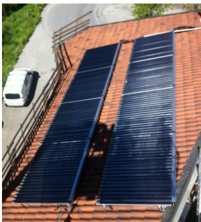
Figure 6 – ETC installed on the roof
