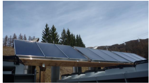
Figure 4 – FPC installed
