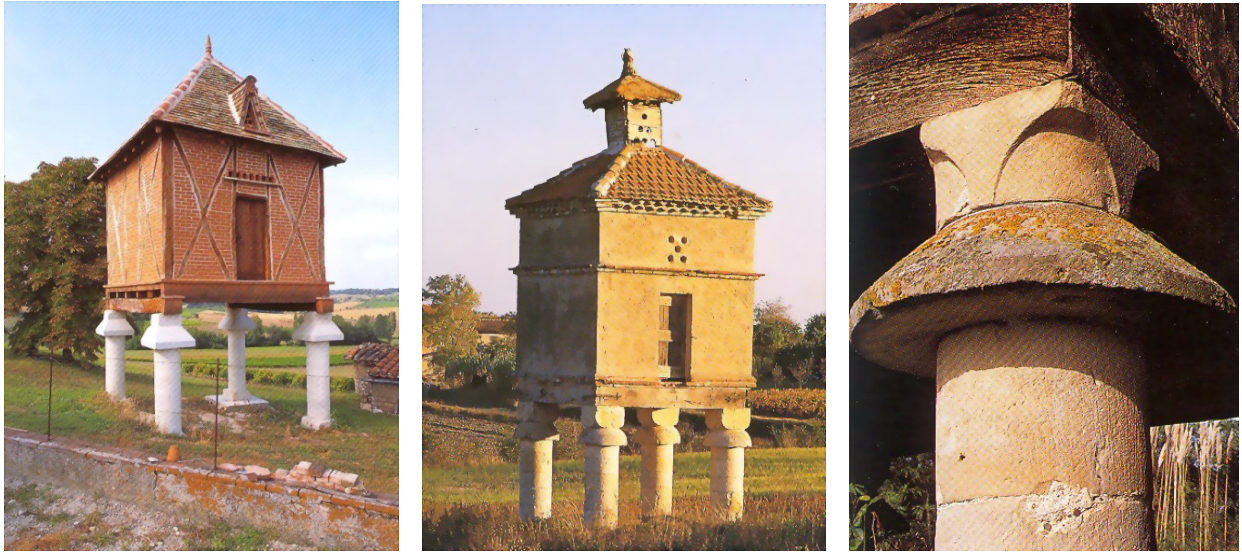
Fig. 1, 2, 3. Midi Pirennais: examples of "pigeonniers" and the particular of a stone pillar
